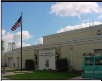
Filtration Plant on North Lake Street
