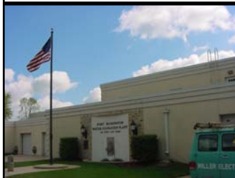
Filtration Plant on North Lake Street
